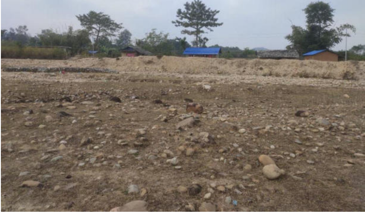
Photo: Existing earthen embankment to mitigate flood risk
