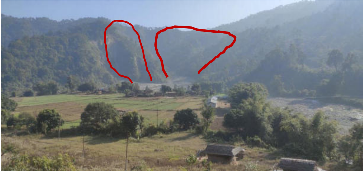
Photo: Landslide and gully erosion site at Hattidhunga
