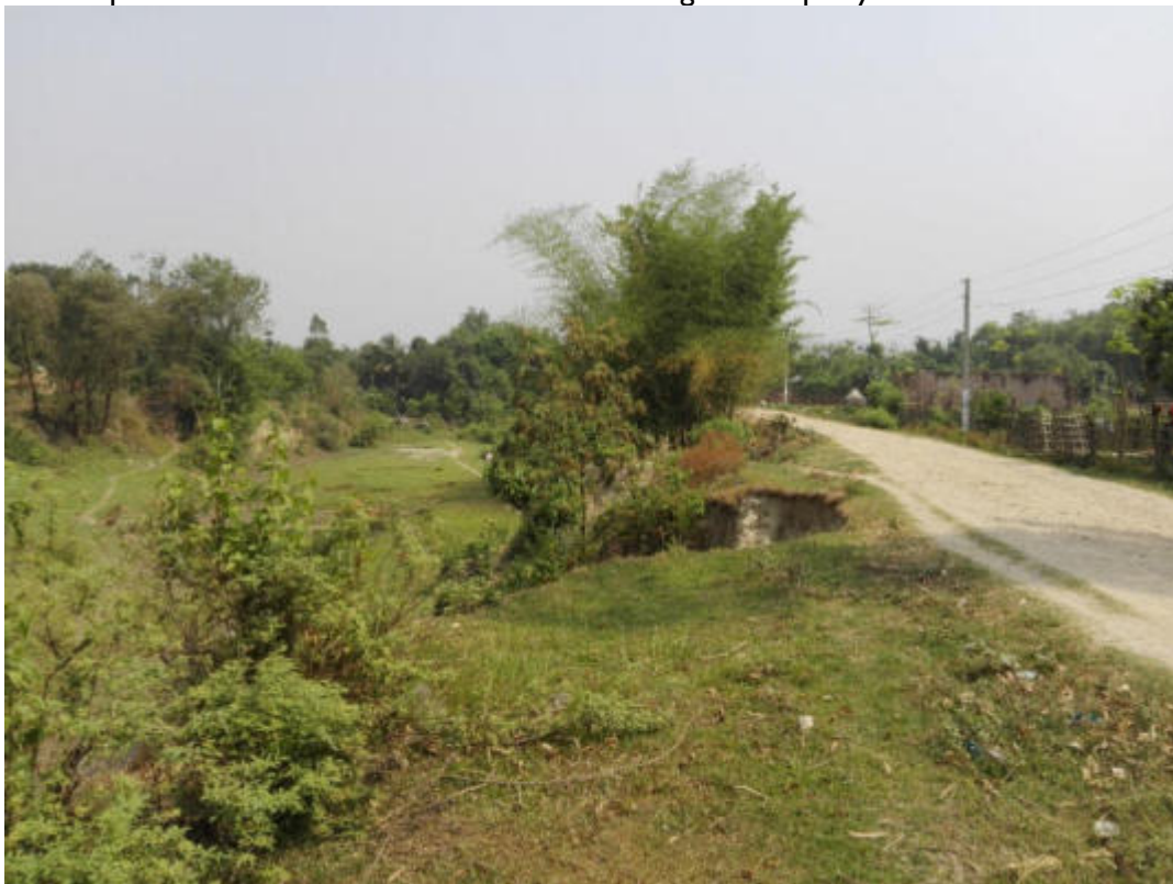
River bank stabilization (26.657276/86.566036) Surunga Municipality-4
