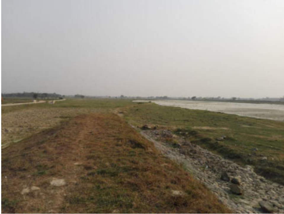
Potential for agroforestry with River bank stabilization (26.518171/86.785266) Rajbiraj Municipality-15
